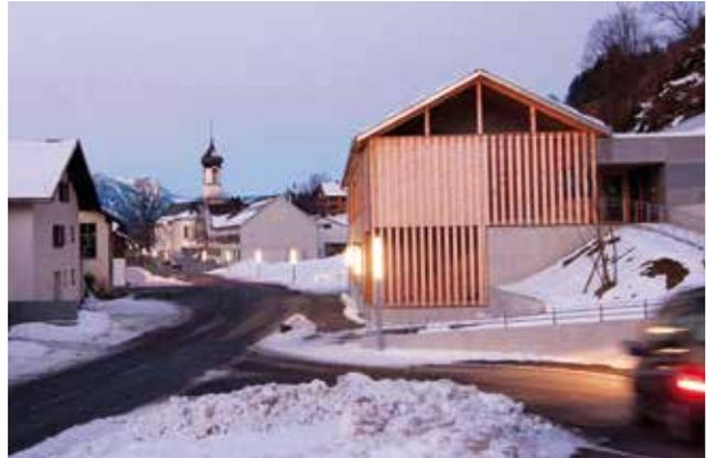
The ceilings were joined to achieve appropriate spans. Outer walls were built with stacked-wood panels, arranged vertically and held together with dowelled pine using no glue. The interior used an application called "pinstripe timber", which was developed and patented by Kaspar Greber. The wood is exposed and untreated.
